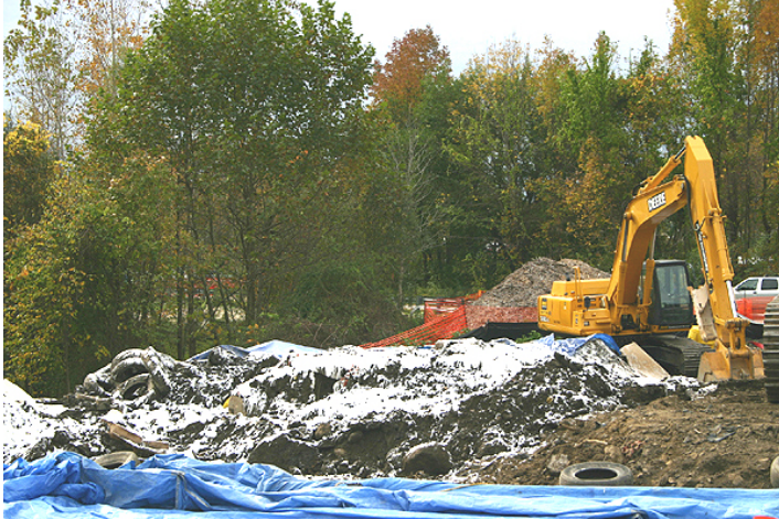
Ringwood Superfund site clean-up. Photo/EPA web site
